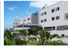
Rudrapur Plant (Green Building)
